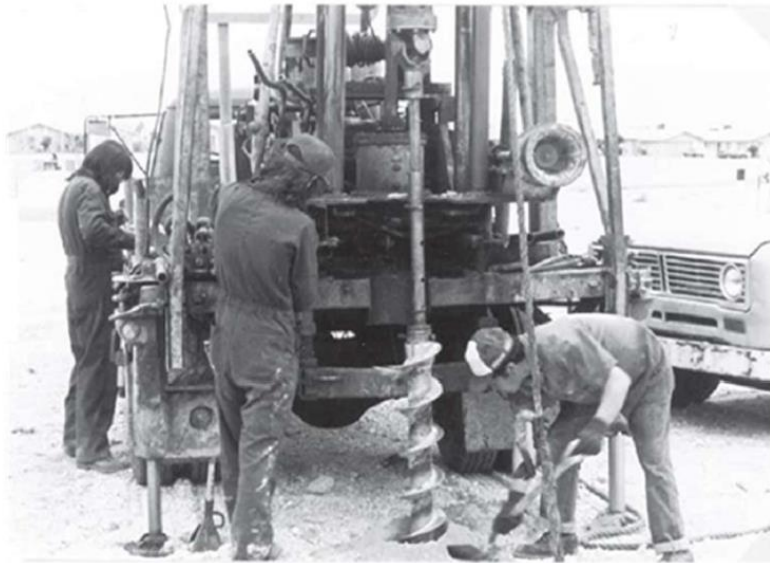
Figure 3-3 Soil drilling using a continuous-flight auger .
