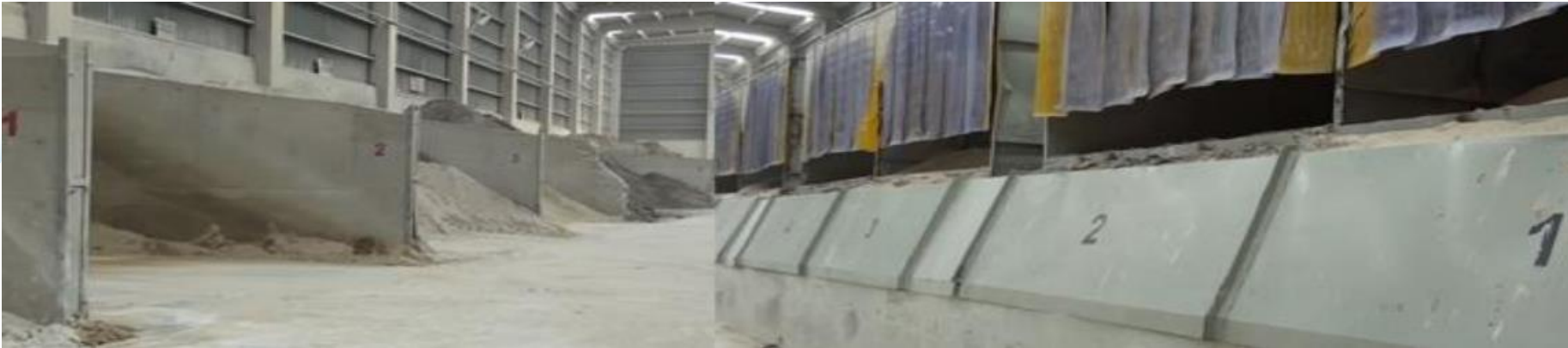
1) Stock Yard; (2) Specific Storage for Batching
