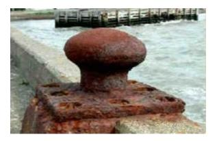
2. **PITTING CORROSION:** Pitting is dangerous because it can lead to failure of the structure with a relatively low overall loss of metal.
