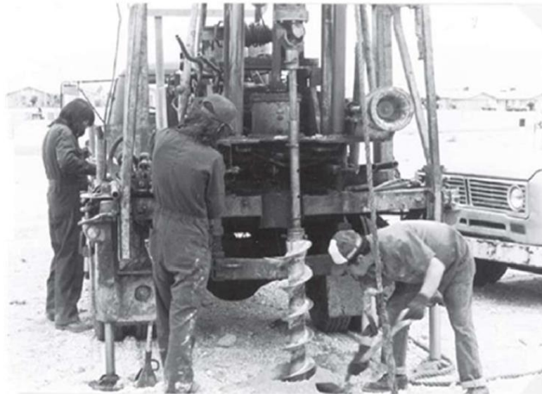
Figure 3-3 Soil drilling using a continuous-flight auger .
