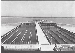
The settling tank is designed so as to remove the settled water from the tank without carrying away any of the floc particles. In ideal sedimentation process, the average velocity of the water is equal to its flow rate divided by the area through which it flows:
