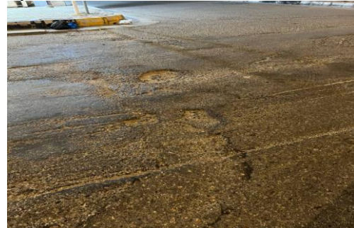
:Alligator Cracking (or Fatigue Cracking)
