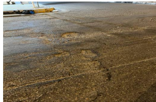
:Alligator Cracking (or Fatigue Cracking)
